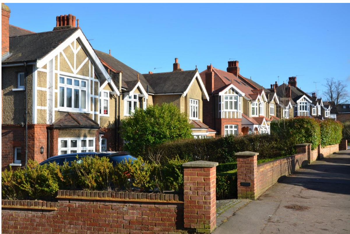
A row of houses built in the second development stage of Hadley Wood between 1897 and 1914
